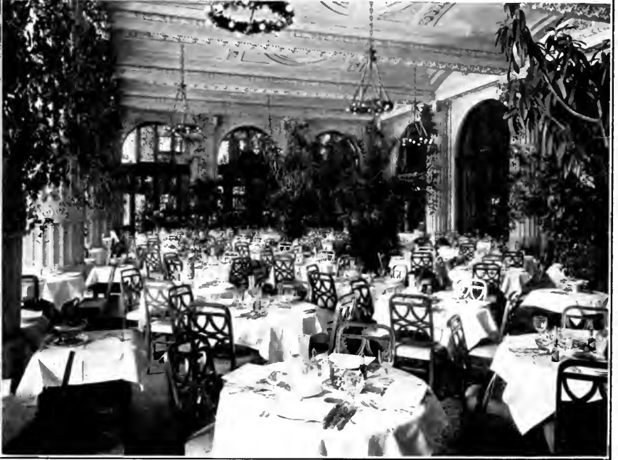
THE RESTAURANT AND THE PALM-ROOM OF THE HOTEL BELLEVUE-STRATFORD. Philadelphia, Pa.
